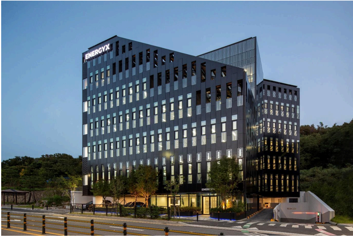
EnergyX DY-Building, a plus-energy building achieving an energy self-sufficiency rate of 122% in South Korea | Photo courtesy of EnergyX
